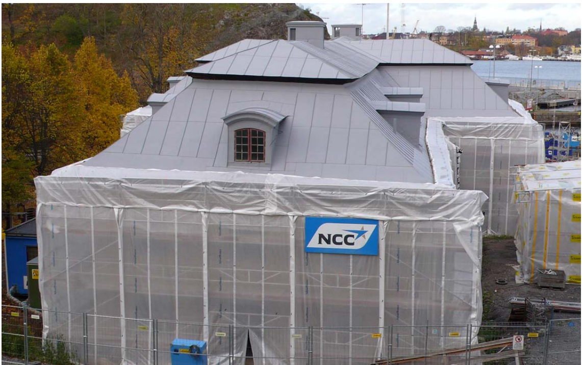
Tak under restaurering. 2008-10-27
